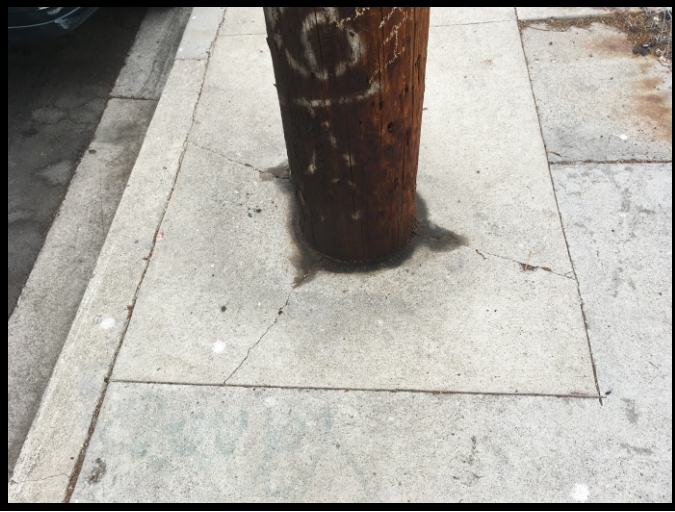
Photo #7: View of staining on concrete at base of pole-mounted transformer.
